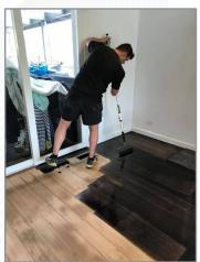
The floor was prepared in the usual way, stained with Urethane Coatings Black Stain added to Urethane Coatings Reducer/Extender. Once dry, two coats of Urethane Coatings Monothane 45 Gloss were applied, followed by a final coat of Urethane Coatings Monothane Satin.
