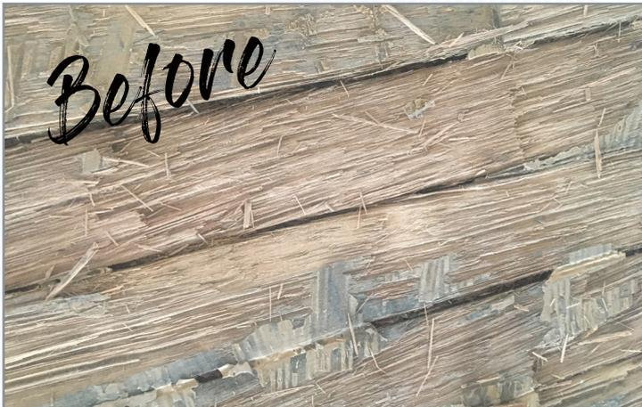
To bring this Tallowwood Floor back to life the floor was sanded and prepared then coated using a Urethane Coatings system of **TIMBERSEAL** and **MONOTHANE SATIN**. The first coat of **TIMBERSEAL** was followed by two coats of **MONOTHANE SATIN**.
